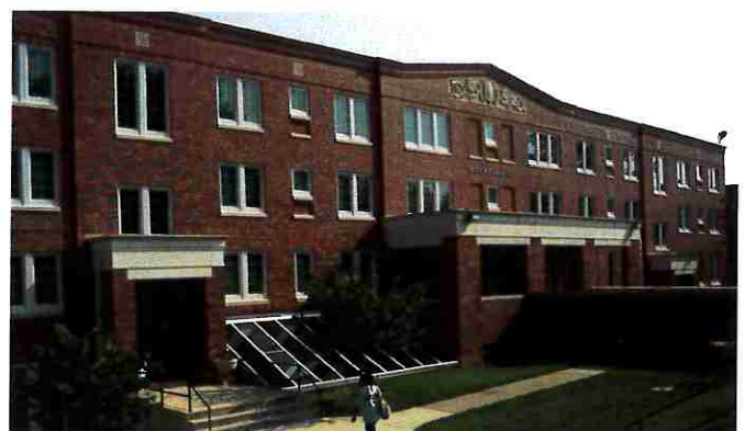
SHSU BELVIN-BUCHANAN HALL AFTER REHABILITATION
