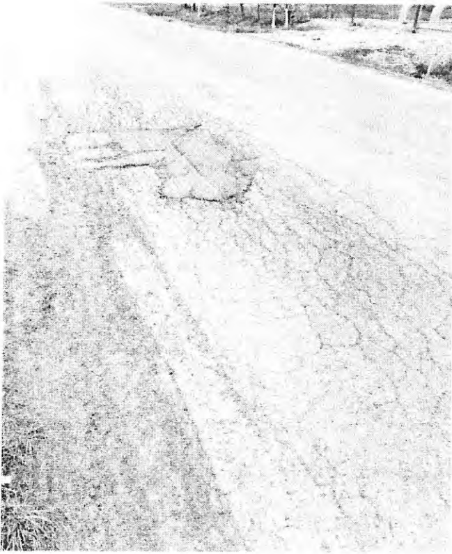
Erie St - (P-9) - Damage Roadway - (01-07-2022) DN
