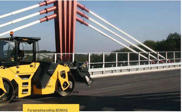
tandem rollers with TanGO oscillation. Careful compaction on seams & bridges.
